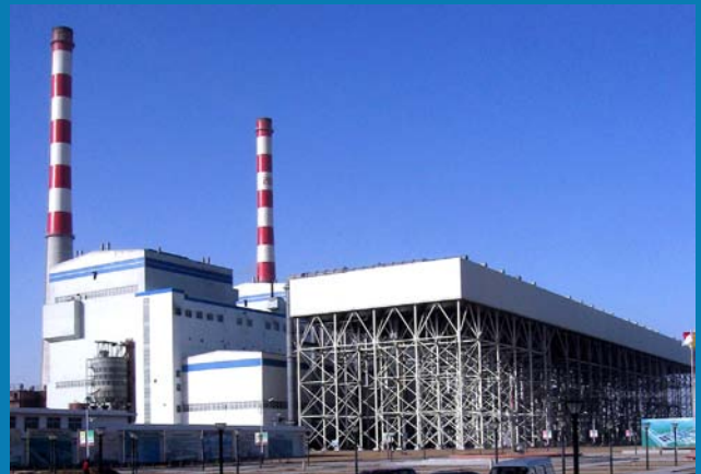
690t/h 循环流化床燃煤锅炉
